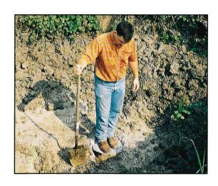
Step 6: Backfill the area around the top of the cutoff casing with clean native soil shaped to a slight mound to direct surface flow away from the site.
