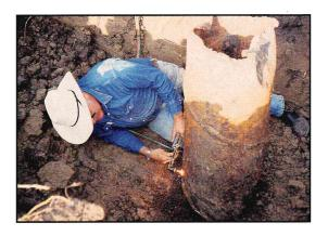
Step 2: Remove sufficient soil from around the casing to allow the casing to be cut off 3 feet below the land surface. Cut off exposed casing.
