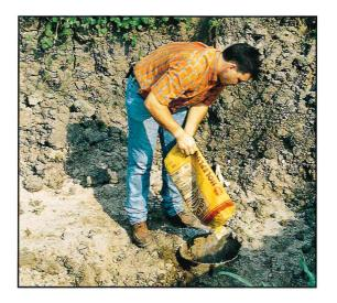
Step 5: Fill the casing with a clean sand and gravel mix to at least 10 feet above the top of the screens and 20 feet below the ground surface (30 feet of the surface if there are underground storage tanks at the site). Fill the remaining space with granular or chip bentonite. (See Table 1 for amounts of sand/gravel mix and bentonite.)
